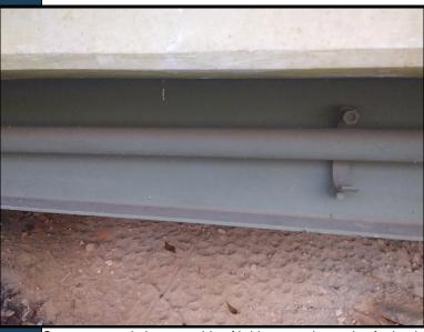
Green on metal pipe east side of bridge tested negative for lead-8 based paint.
