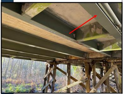
Green on metal beams tested negative for lead-based paint.
